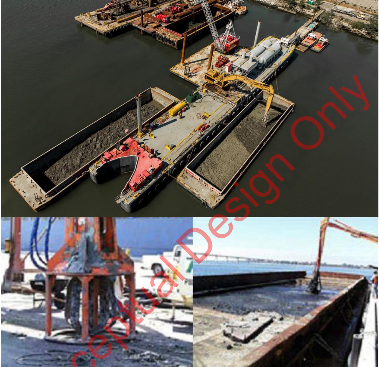
Figure 1-6: In- Barge Stabilization Operation and Typical Mixing Attachments
