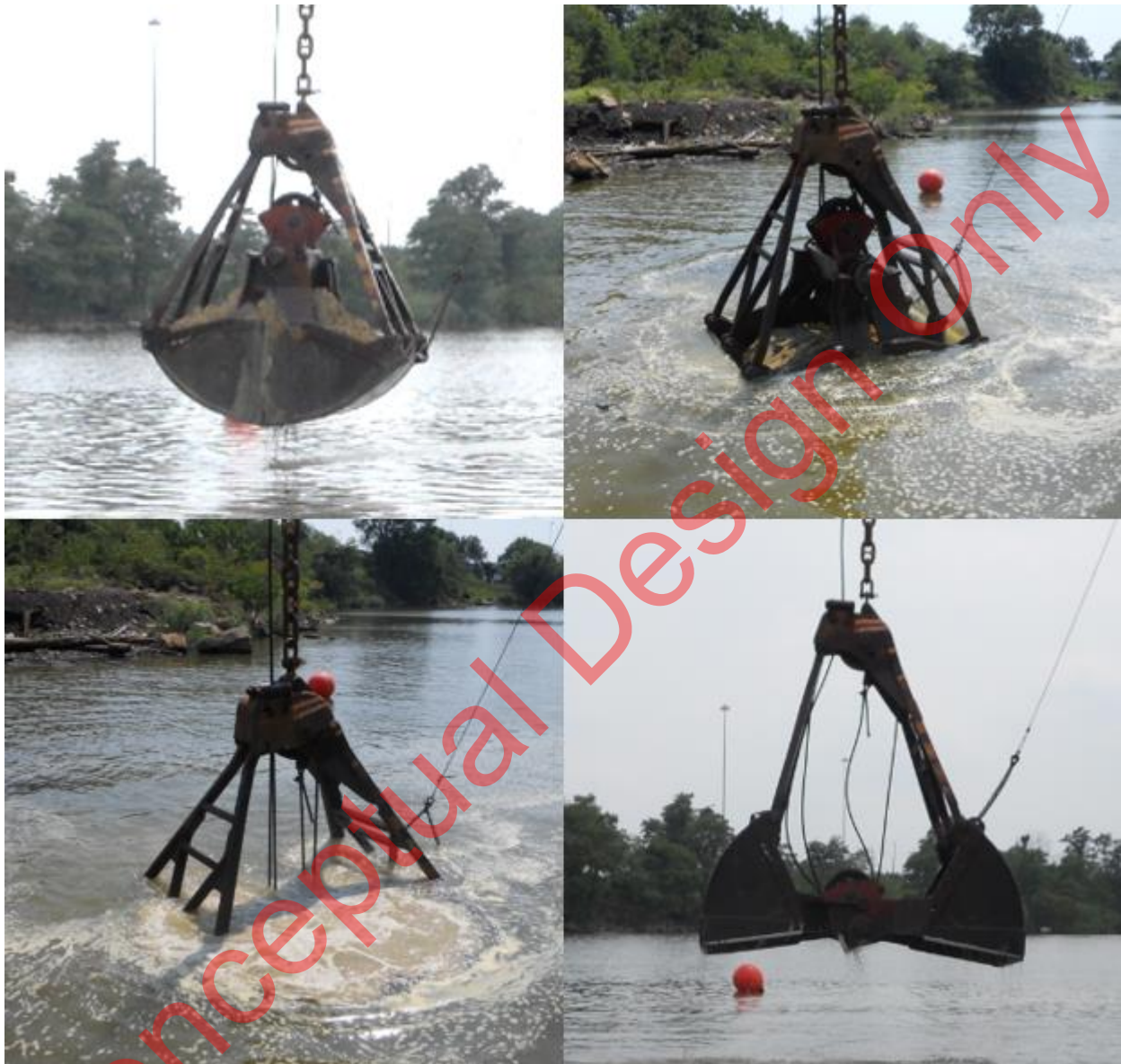
Figure 1-9: Sand Capping Underwater Using Clamshell Bucket
