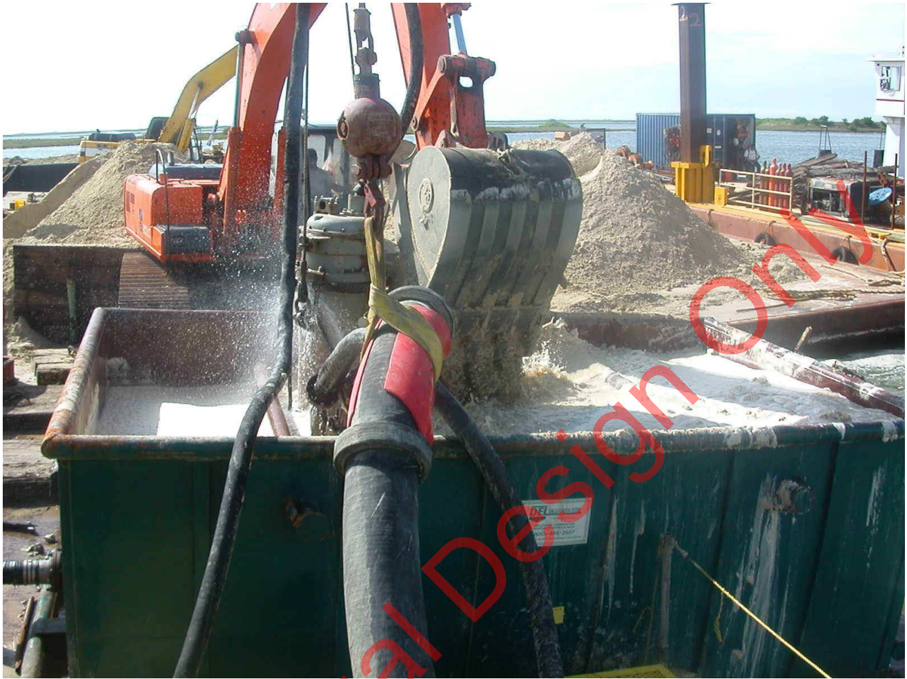
Figure 1-10: Hydraulic Sand Unloading Operation from Land-Based Containment Box
