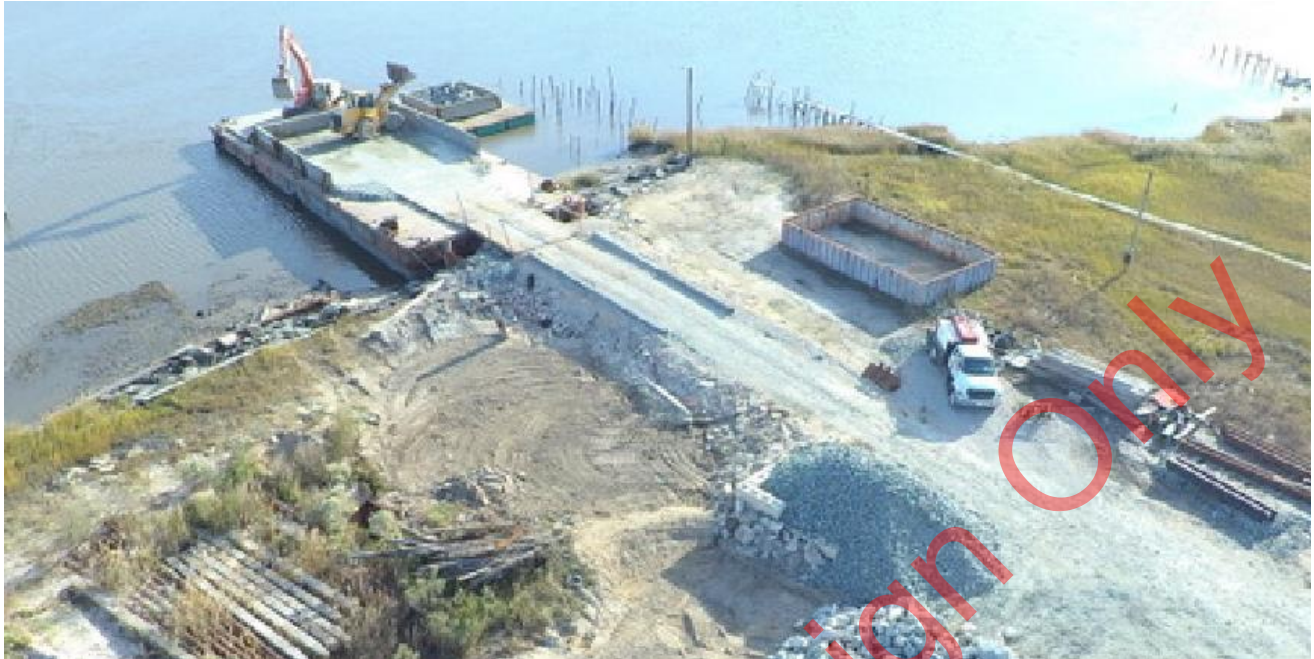
Figure 1-7: Barge Unloading Operation and Stockpile Area
