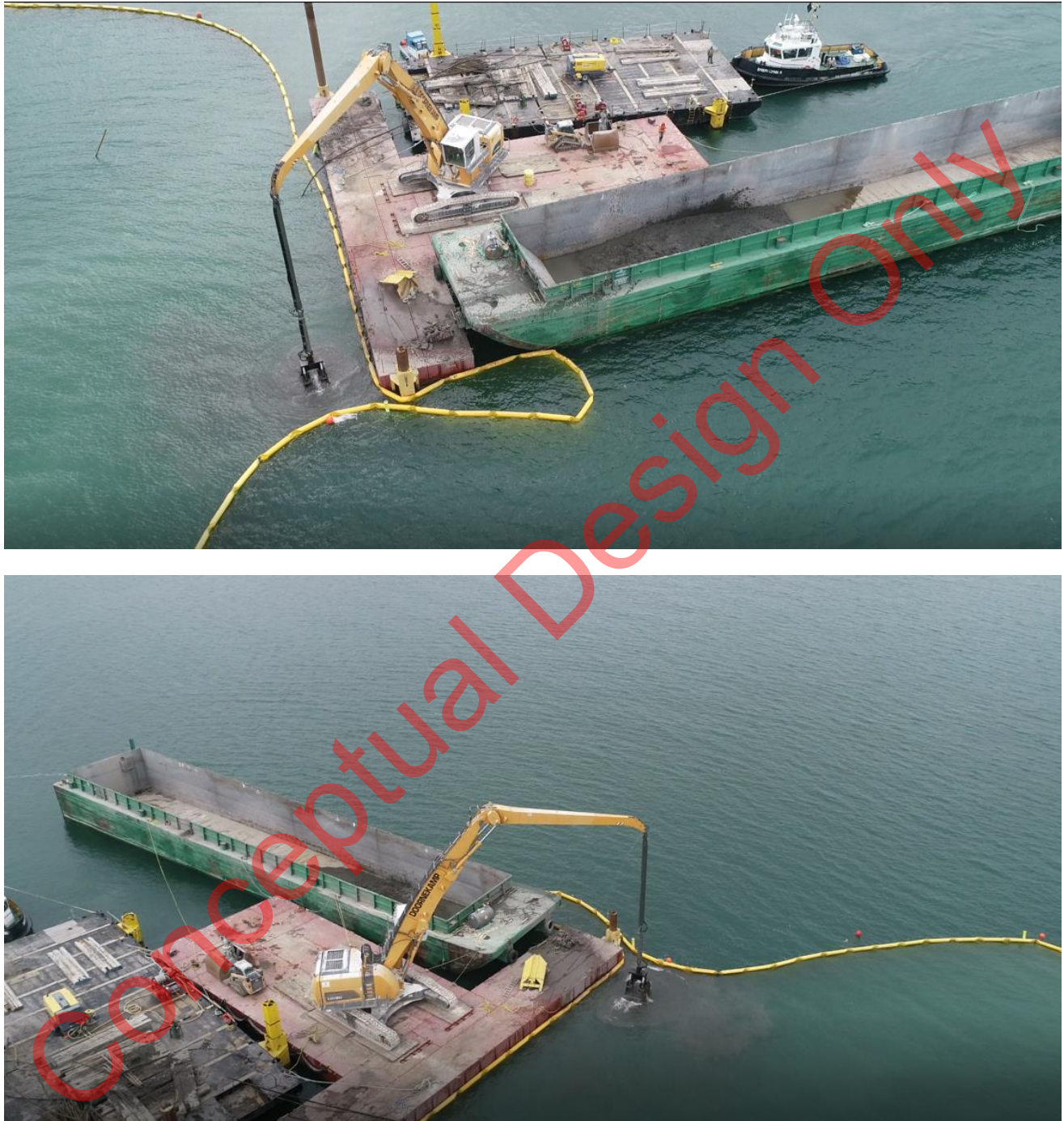
Figure 1-5: Mechanical Dredging Inside Turbidity Control Curtain
