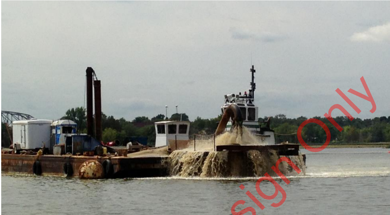
Figure 1-14: Sand Spreading by Pumping through Steel Grate
