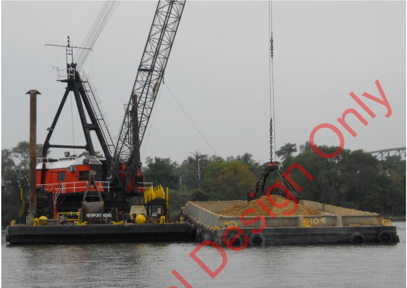
Figure 1-8: Sand Barge Unloading Operation Using Clamshell Bucket
